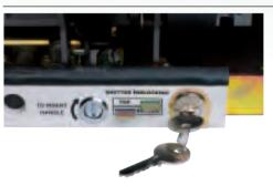
Available for withdrawable circuit breakers only, this sophisticated interlock system secures the circuit breaker in the disconnected position by means of a Ronis or Profalux key. When the key is removed, the safety shutters are automatically locked in position, thus preventing access to the contacts and also ensuring that the racking mechanism is not operable.
