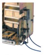
Cable interlocking version shown above available for fixed and withdrawable circuit breakers.
